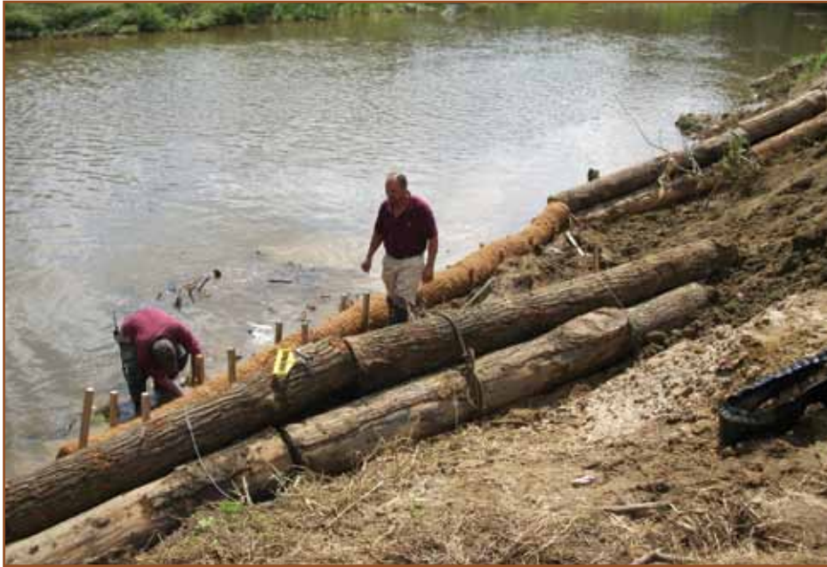
Placement of stunted log vanes and bank toeing (the bank structure) that was covered with lifts of soil.
