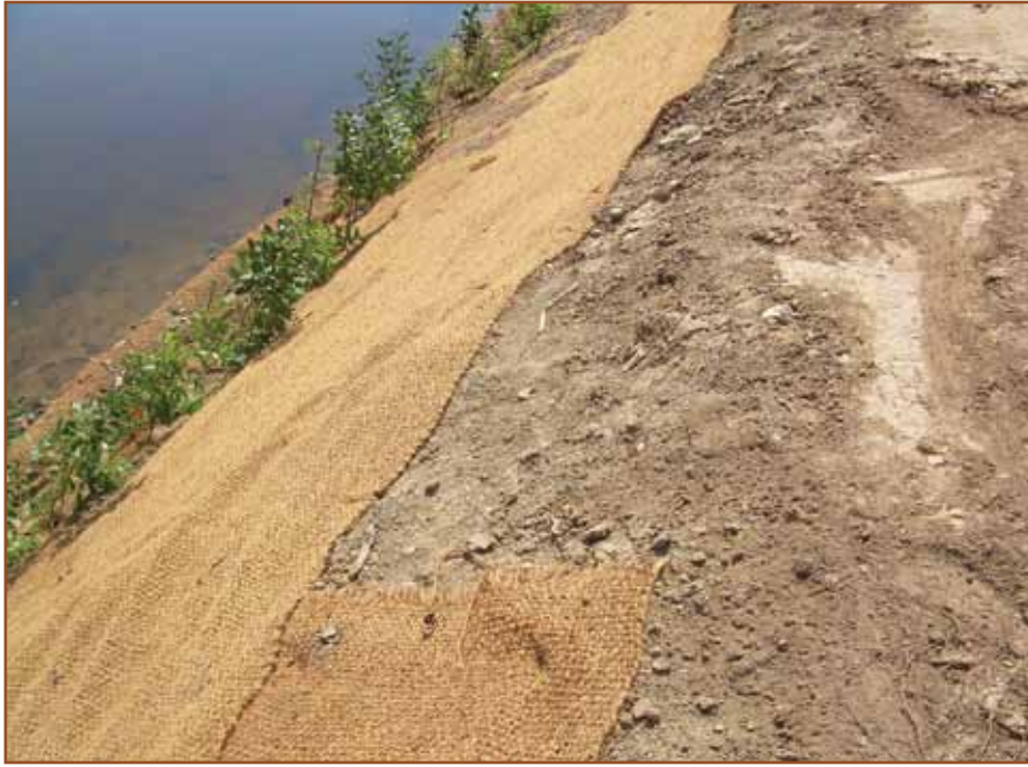
A closer view of the jute mat, which was seeded and stapled down.
